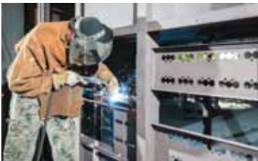
Our Switchboards are designed and fabricated in house.
